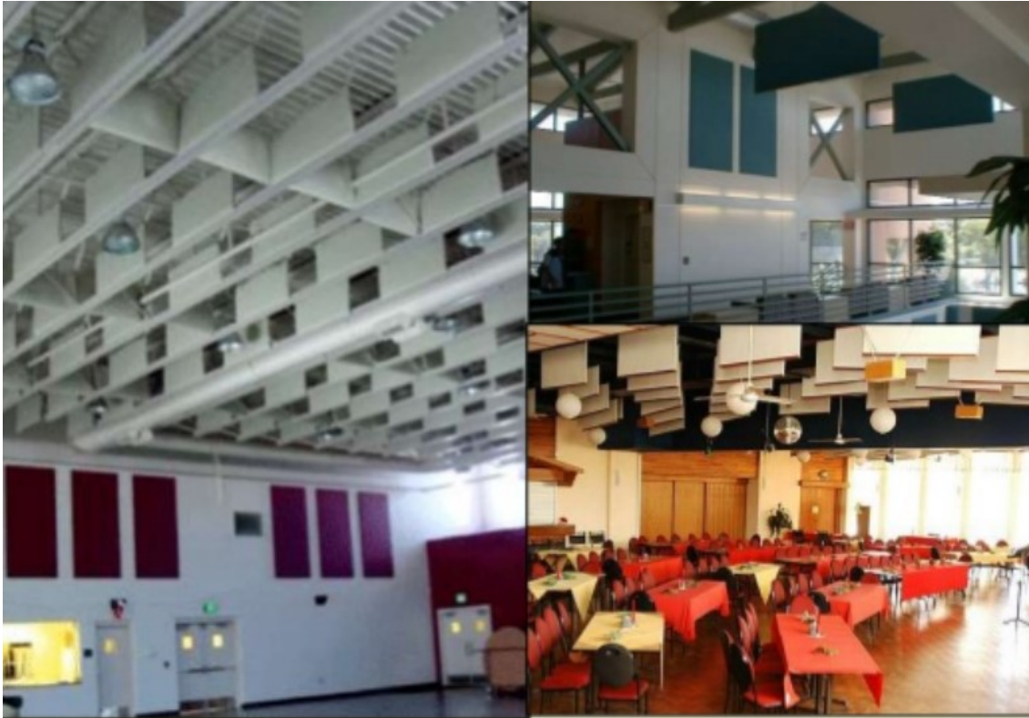
Geocoustic Tiles- special prefabricated units for random application on walls and ceilings.
