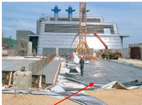
Geomembranes Made Using Polypropylene
