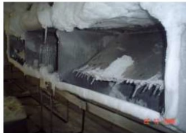
Fig 2. Frost on a duct of a refrigerating unit in a cold store
