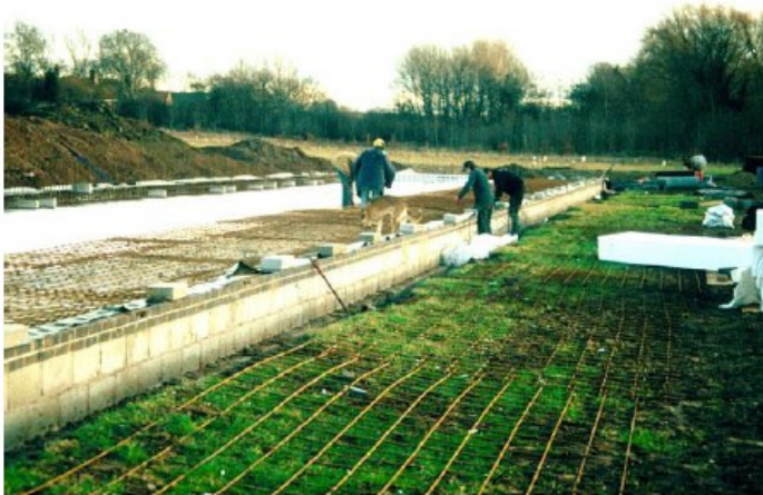
In-situ concrete flooring on 300mm of Expanded Polystyrene insulation.
