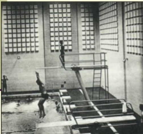
Geocoustic Tiles- special prefabricated units for random application on walls and ceilings.
