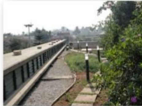
Trombe walls help in insulating the hostels
