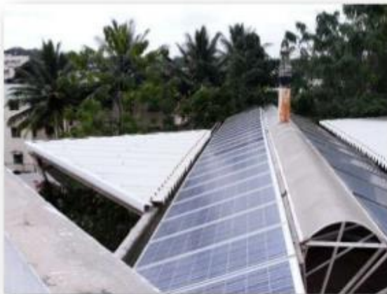
Solar Photovoltaic integrated with the roof provide natural light and electricity
