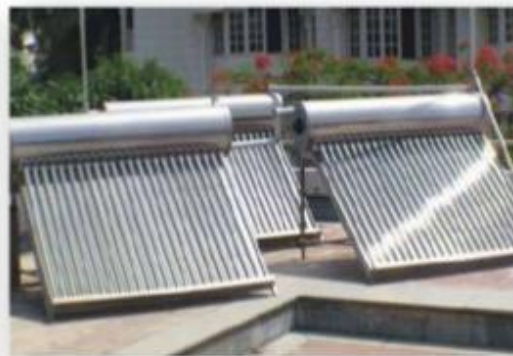
Solar water heaters which meet the hot-water requirements of the campus
