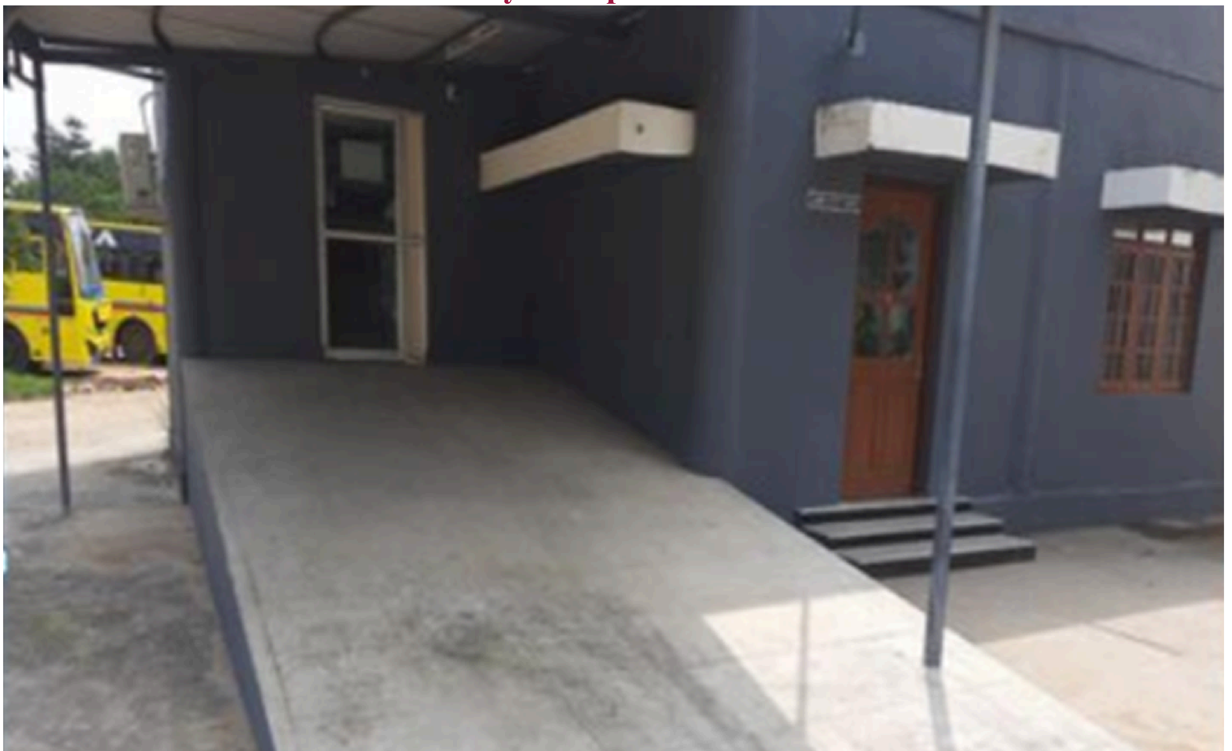
Accessible Facility at Sathyabama Indoor Stadium
