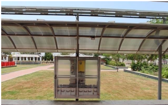
Figure 23 Solar panels with controller
